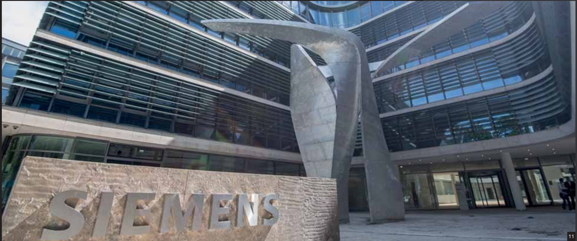
Siemens Headquarter, Munich/Germany
